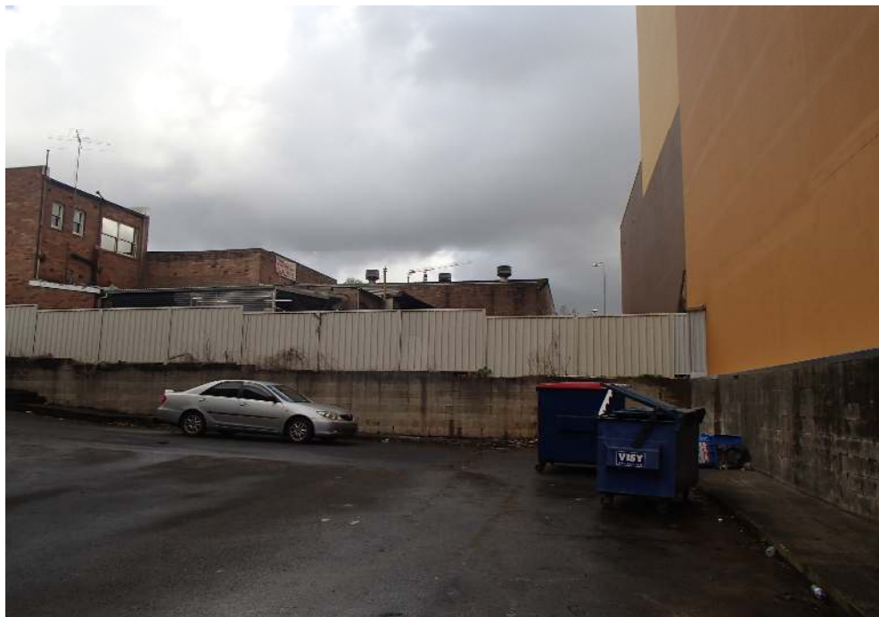
Photograph 6 (2016) - Looking West from Loading Dock Towards Car Service Centre/Mechanic
