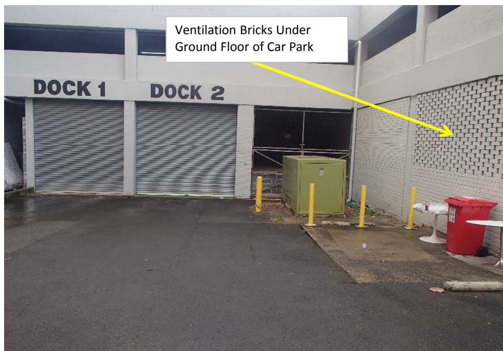
Photograph 7 (2016) - Looking East Towards Loading Dock
