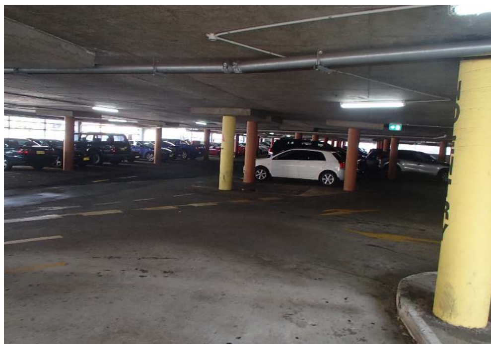
Photograph 8 (2016) - Looking West Across Ground Floor Car Park
