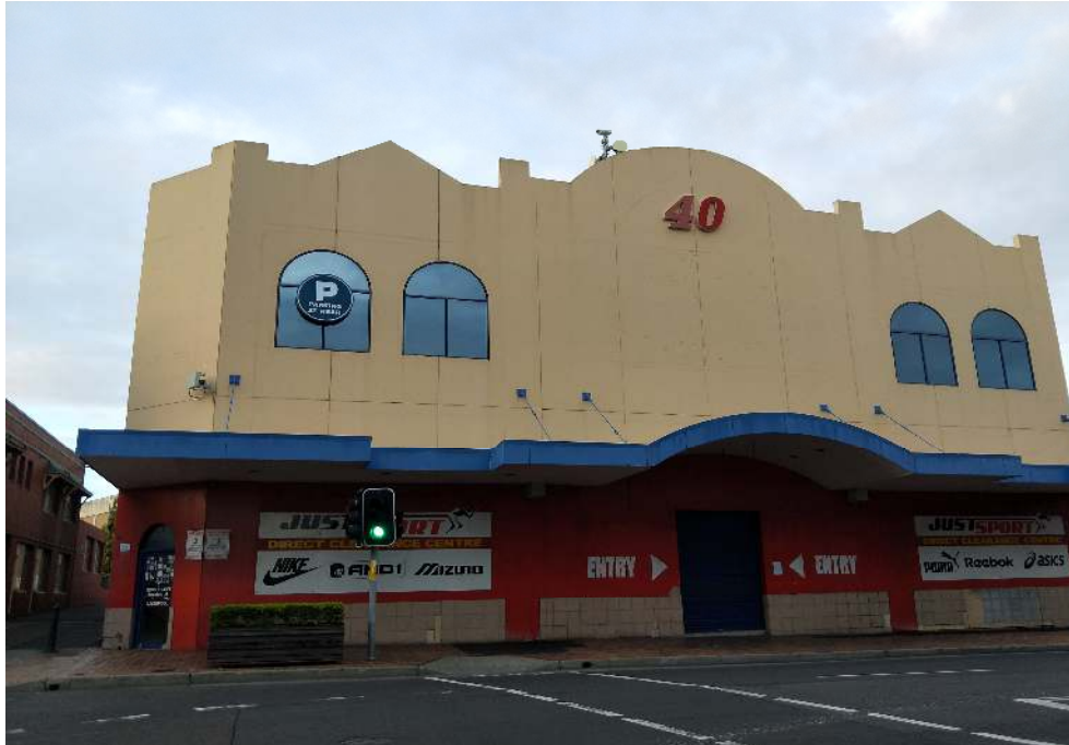
Photograph 13 (2019) - Sports shop located on the north eastern corner of the site.
